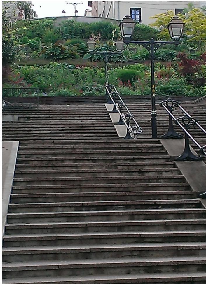
Figure 6: New staircase and garden, Crêt de Roc
